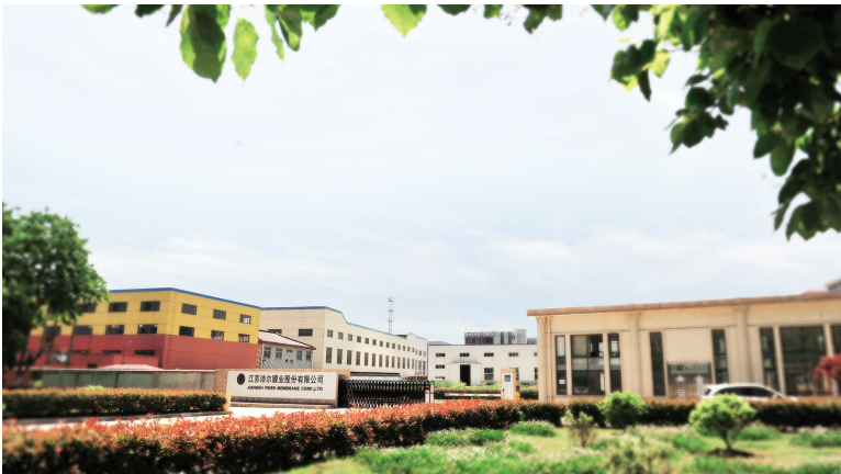
Peier Membrane Production Base
